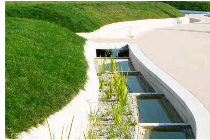
Channels alongside walkways to convey water on the surface
